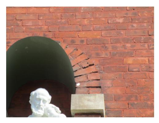
Photo 7 - Brick Masonry Deterioration, 2017
