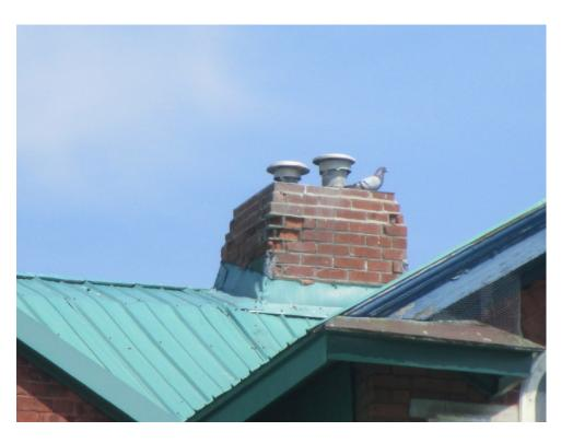
Photo 9 - Chimney Masonry Deterioration, 2017
