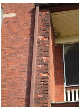
Photo 5 – Brick Masonry Deterioration, 2017
